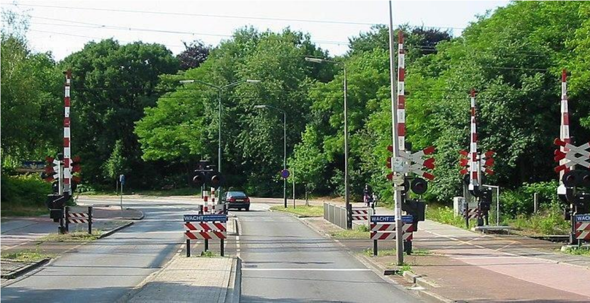
Fig 8. Segregated Road and Cycleway level crossing at Amersfoort Netherlands. All barriers operated simultaneously by one control system. Such systems are common in the Netherlands and Scandinavia.
